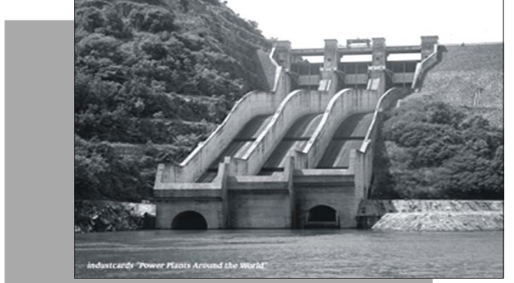
Industrially 'Power Plants Around the World'
